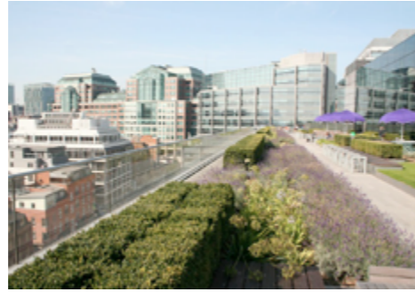
Green Roofs Green roofs can increase the thermal mass of a building, absorbing solar energy through the day and releasing heat at night.
