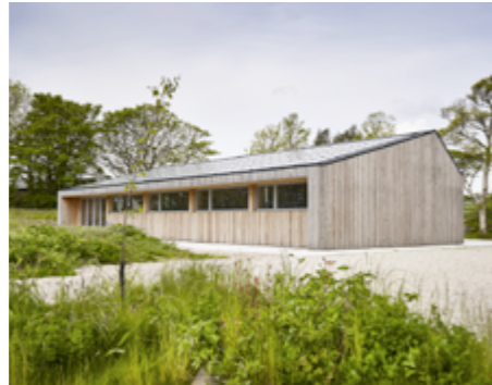
Argal Workshops (Gluckman Smith) A Cornish former farmstead, previously derelict, was transformed into rural workshops for a local furniture and product designer, to Passivhaus standards, making a new working community for the area.
