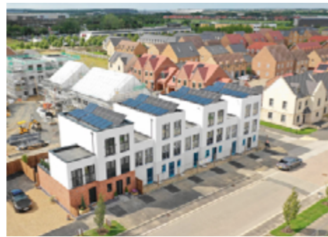
Project Etopia, Corby Uses combined solar PV's and thermal panel to deliver net zero carbon on site.
