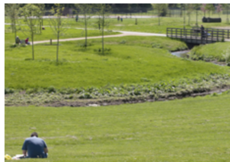
Ladywell Fields, Lewisham (SuDS) Designed to create more sustainable drainage and reduce flooding, the river channel was modified to create a naturalistic setting incorporating backwaters and wetlands.
