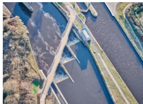
Flood Management Knothrop Weir (Leeds) provides an echelon of three new pneumatically moveable weirs that can be lowered to let floodwater discharge quickly downstream; and a shared foot and cycle bridge
